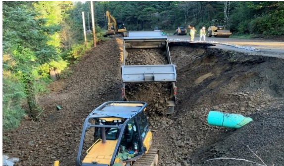
Rock Armoring for New Slope
