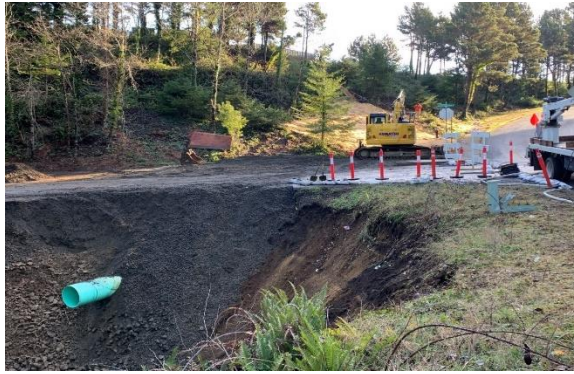
Complete 24" Storm Repair Across Oceanview Drive Towards Walmart
