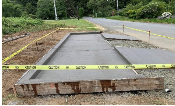
Concrete Pad for Trash Enclosures
