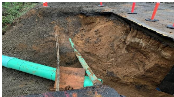
Initial Slide 8" Sewer Pipe Repair
