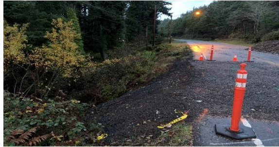
Temporary Slide Repair
