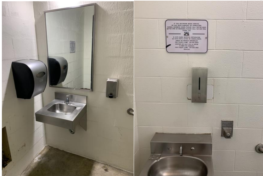
Parks - Restroom Renovations
