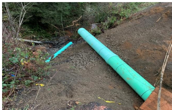
24" Storm Pipe Replacement
