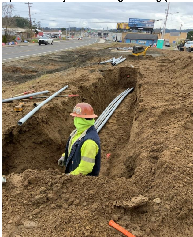
Placing Underground Conduit as Part of Phase 2
