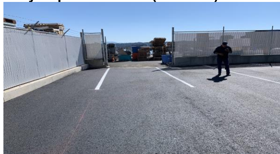
Bay Boulevard Parking Lot Reconstruction
