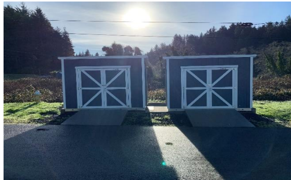
Finished Trash Enclosures
