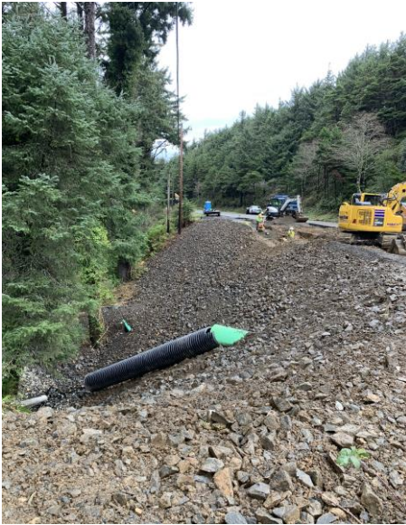
Rock Armoring for New Slope / Final Sanitary Sewer Repair in Progress
