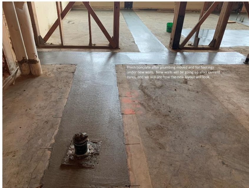
Performing Arts Center Renovation
