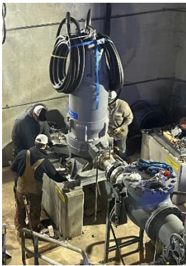
North Side Pump Station Installation
