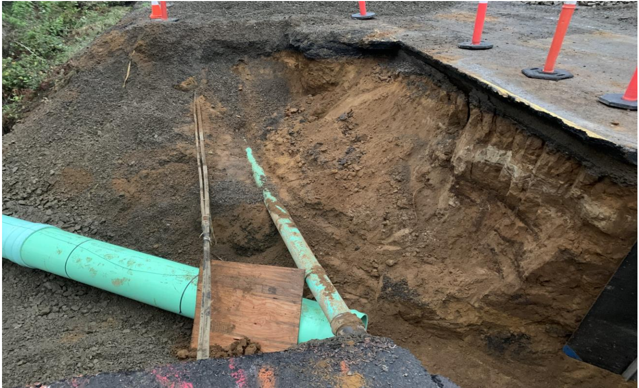
Initial Slide 8" Sewer Pipe Repair
