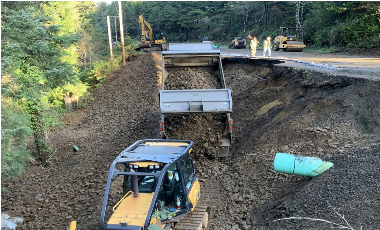
Rock Armoring for New slope
