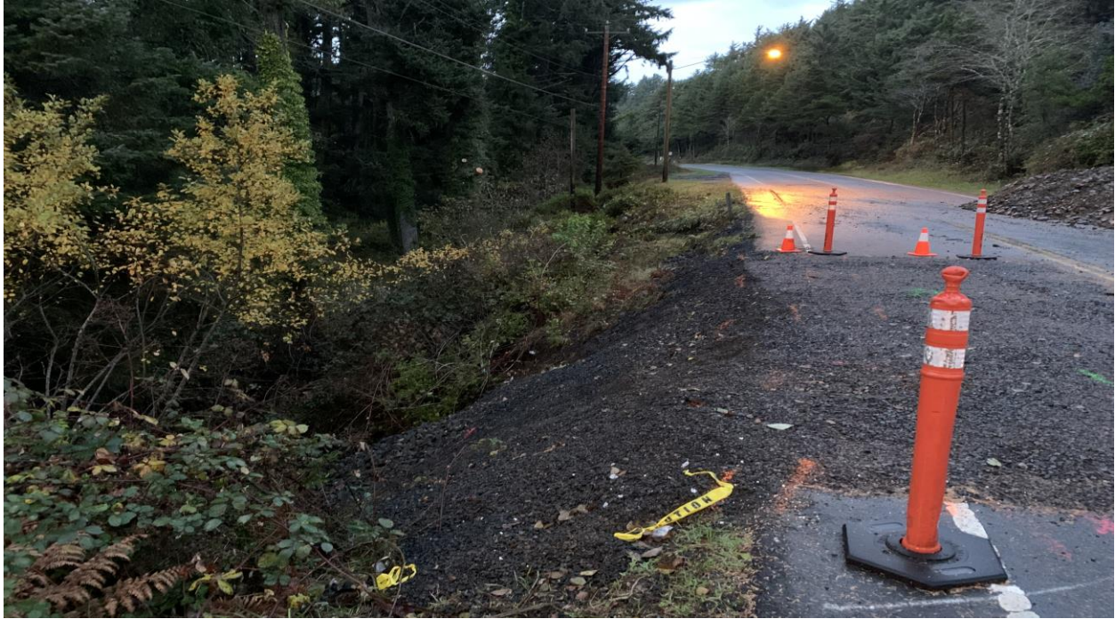
Temporary Slide Repair
