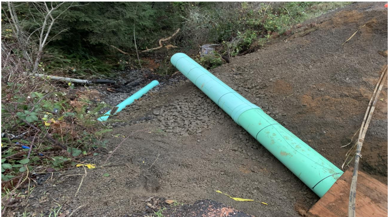
24" Storm Pipe Replacement
