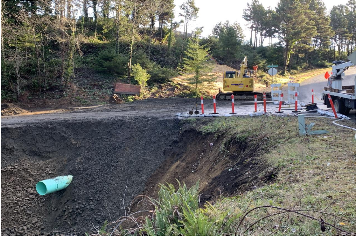
Complete 24" Storm Repair Across Oceanview Drive Towards Walmart
