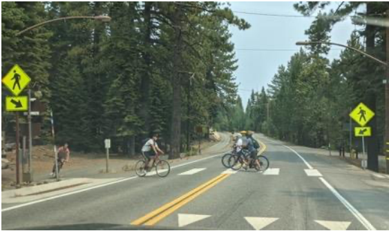
Marked street crossing for multi-use path
