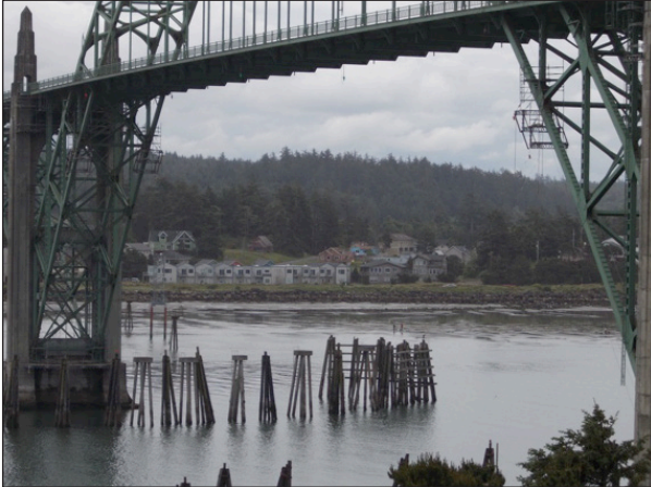
View south under the bridge
