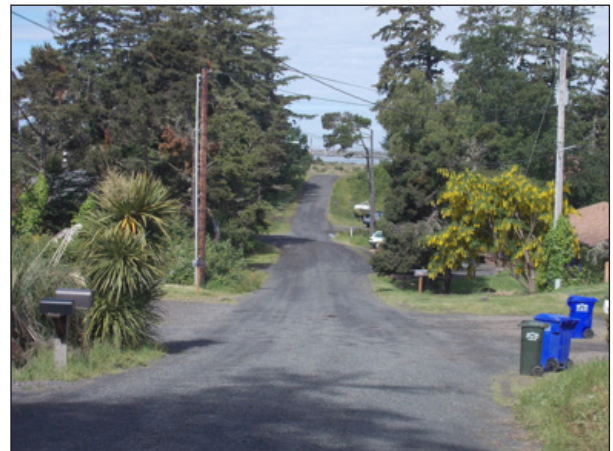
SW 29th Street Looking West
