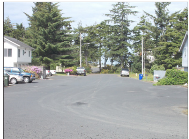
SW 30th Street Looking West
