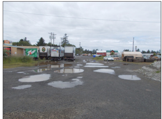
SW 35th Street Looking West
