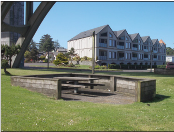
Yaquina Bay Bridge Open Space Looking Southwest
