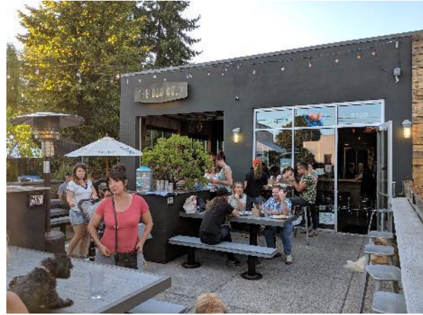
Small restaurant conversion (Portland, OR)
