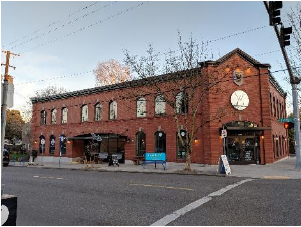
New-construction corner businesses: stores and offices above
