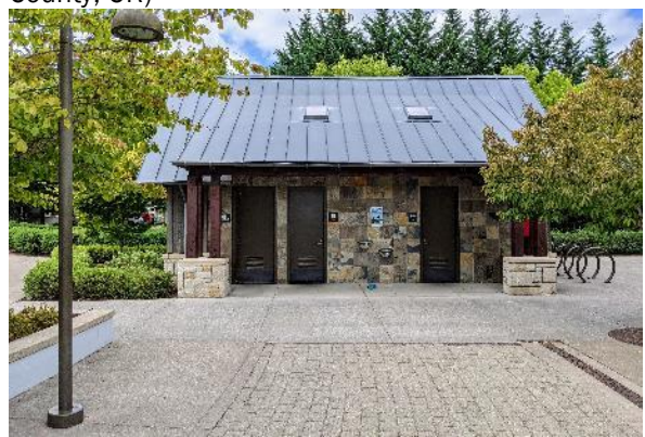
Trail/Park restroom (Foothills Park - Lake Oswego, OR)
