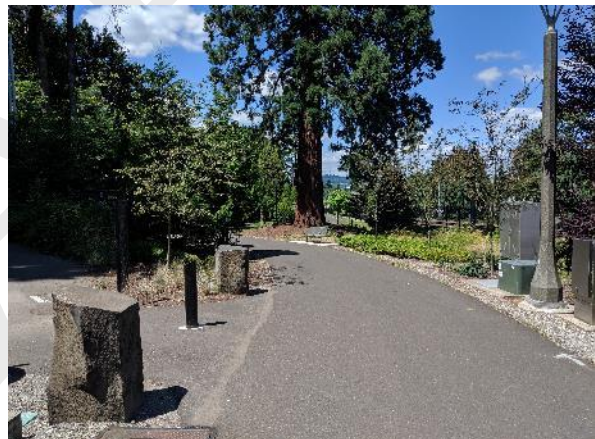
Trail branding with basalt stone, rest area pullouts, and unique lighting fixtures (Trolley Trail, Clackamas County, OR)
