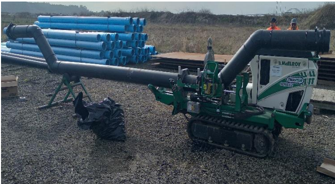
Yaquina Industrial Park Waterline Project
