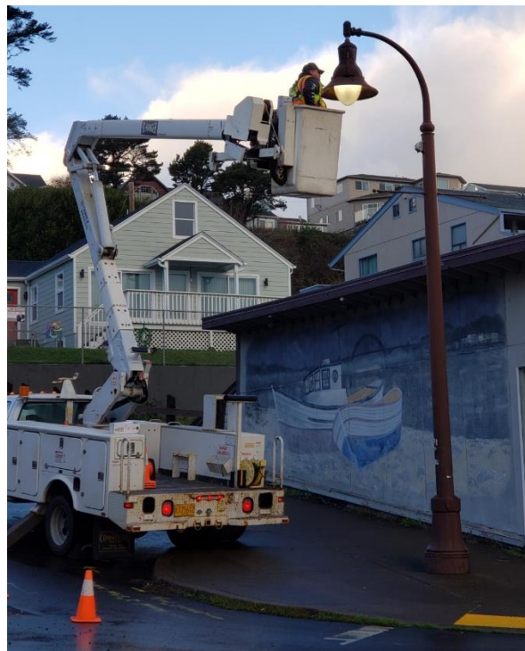
(Facilities Crew Working on Street Light)
