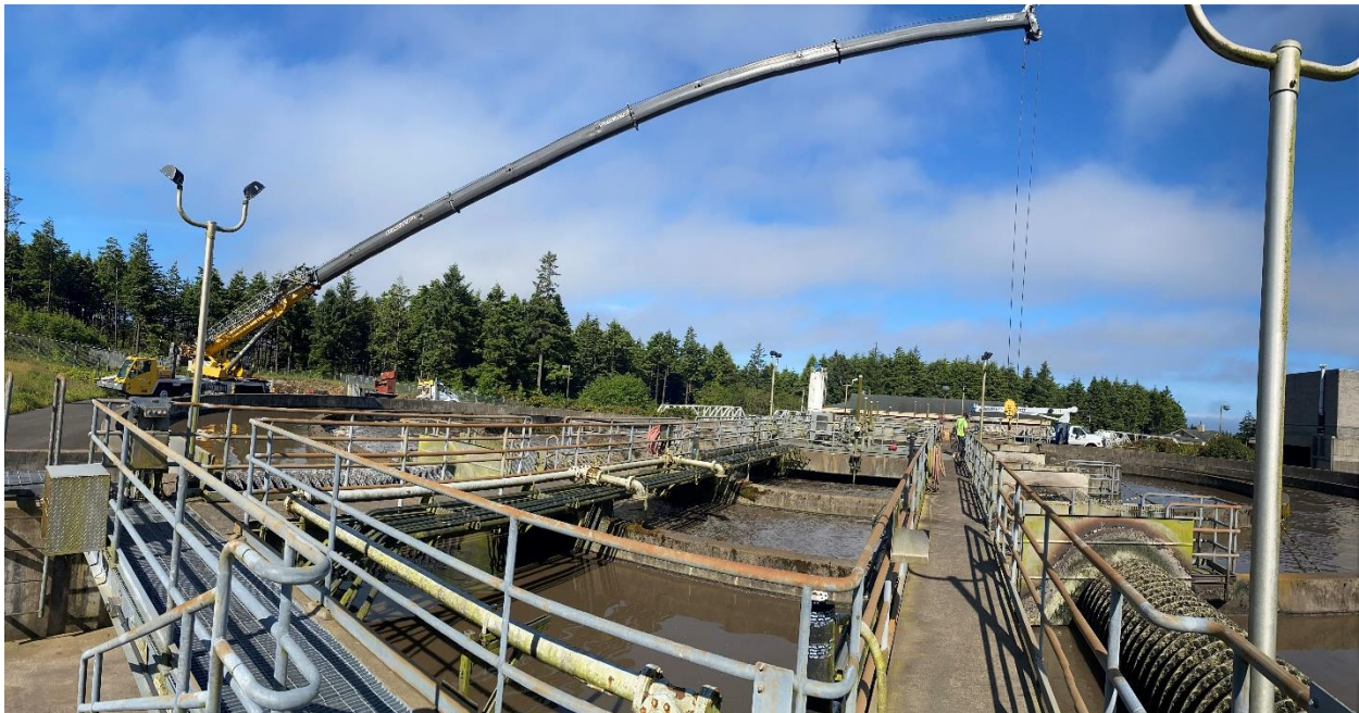
Wastewater Treatment Plant Motor Removal
