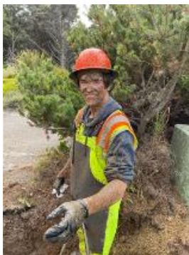
WWC crew using the Jetter
