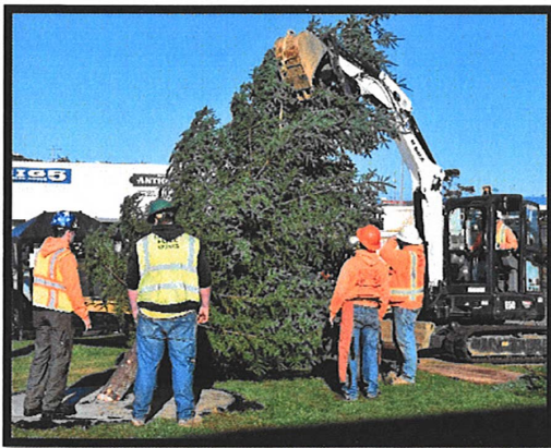
Public Works Tree Installation
