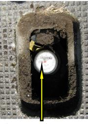
Flip the round lid open to reveal the meter face. Can you see the small red triangle? That's a flow indicator, sensing small flows of water through meter.
