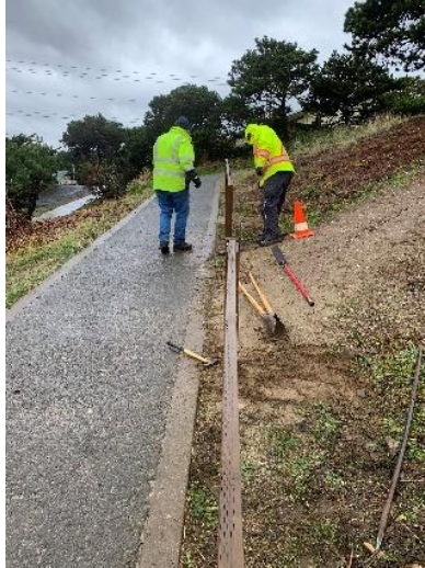
*Fence rails being installed @ Coast Park
