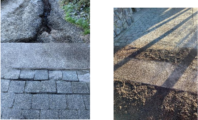
*Beach access repair @ Don & Ann Davis Park
