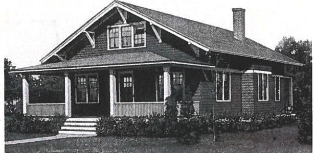
Front gabled roof with hip roofed porch
