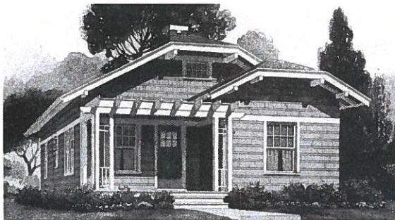
Multiple distinct low pitched gabled roofs (with clipped gables/jerkinhead roof)
