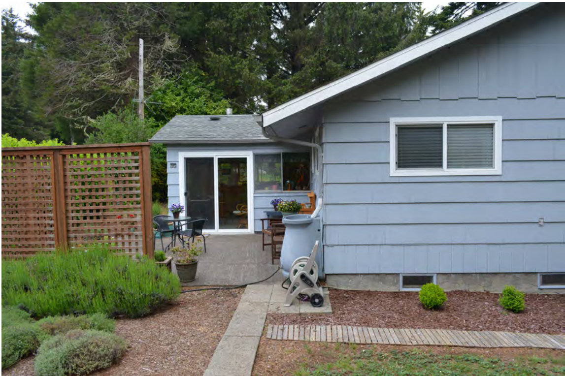
View: Side / east facade with back porch / entrance, view to the west
