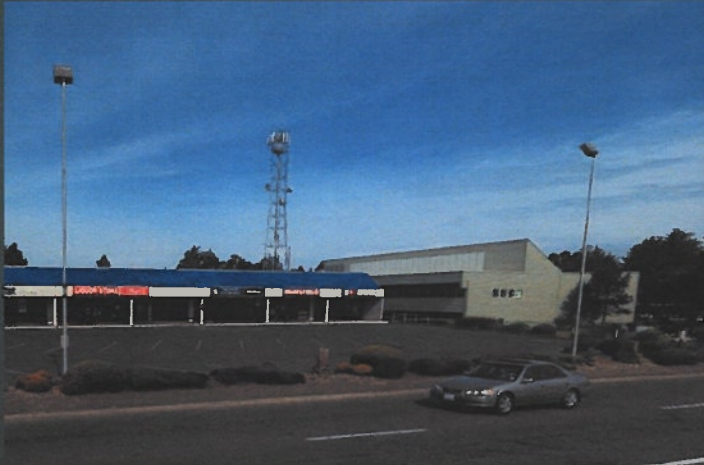
Central Lincoln Lattice Tower
