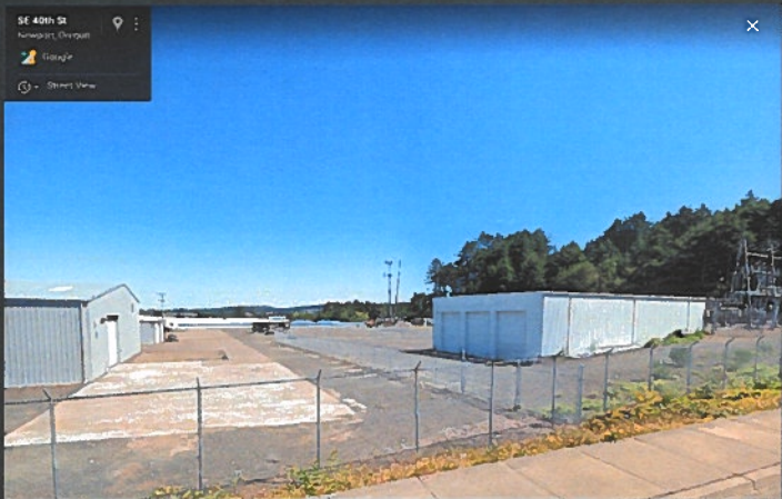
Former PUD Maintenance Site
