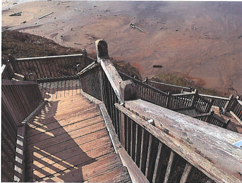
Photo 3: Access Site 3 – Access Structure on Steep Slope
