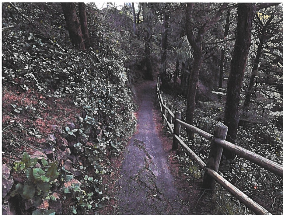
Photo 2: Access Site 2 – Steep Slopes Adjacent to Trail
