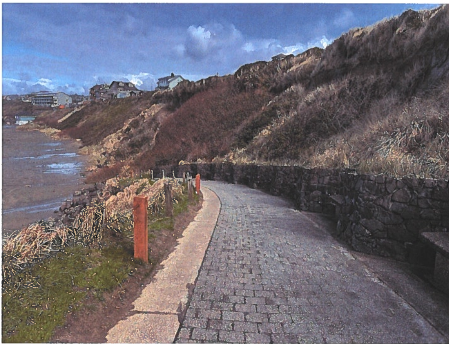
Photo 5: Access Site 5 – Paved Walkway Adjacent to Steep Slope
