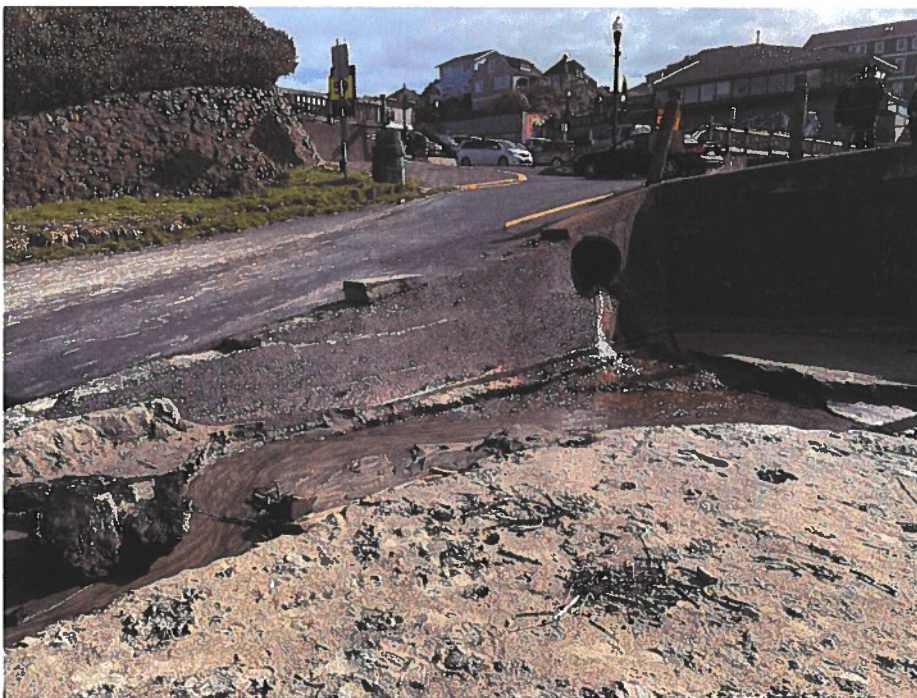
Photo 6: Access Site 6 – Ramp to Beach Adjacent to Retaining Walls
