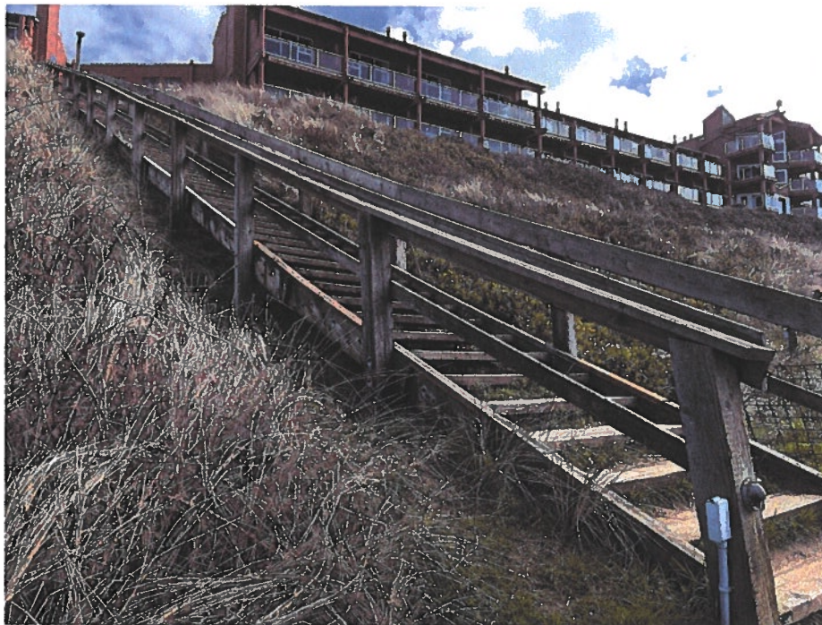
Photo 4: Access Site 4 – Access Structure on Steep Slope
