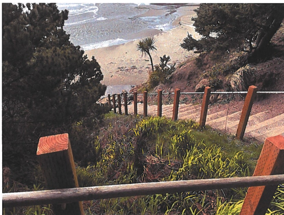
Photo 10: Access Site 10 – Access Along Steep Slope
