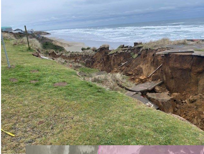
Left: Remnants of a failed condominium foundation at "Jump-Off Joe" a geologically unstable headland north of the Nye Beach neighborhood. (Source: Oregon Coast Beach Connection, 2021)
