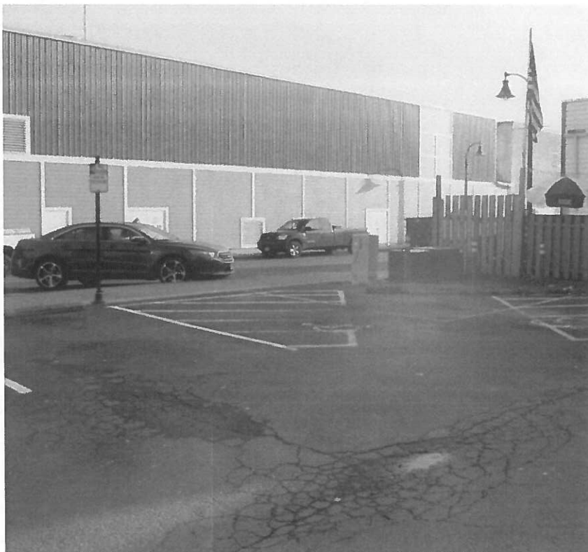
Fatigue Cracking – Abbey Street Lot (2016)
