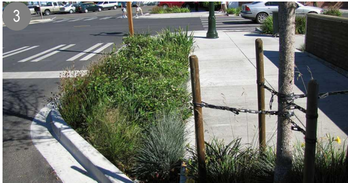
Figure 32. Rain Garden in Port Townsend, Washington Source: The Walc Institute
