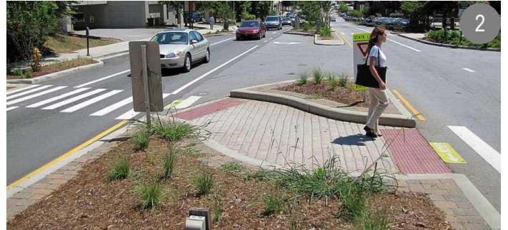
Figure 31. Crossing Island in Asheville, North Carolina Source: The Walc Institute
