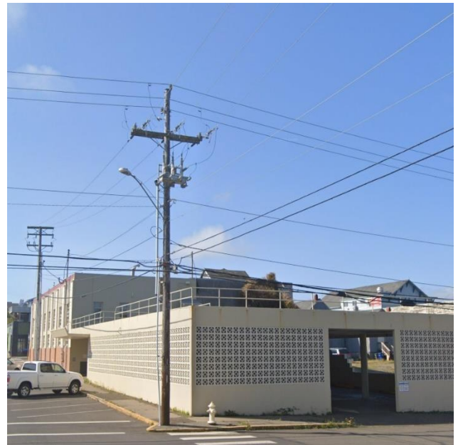
Figure 41. Existing Overhead Utilities
