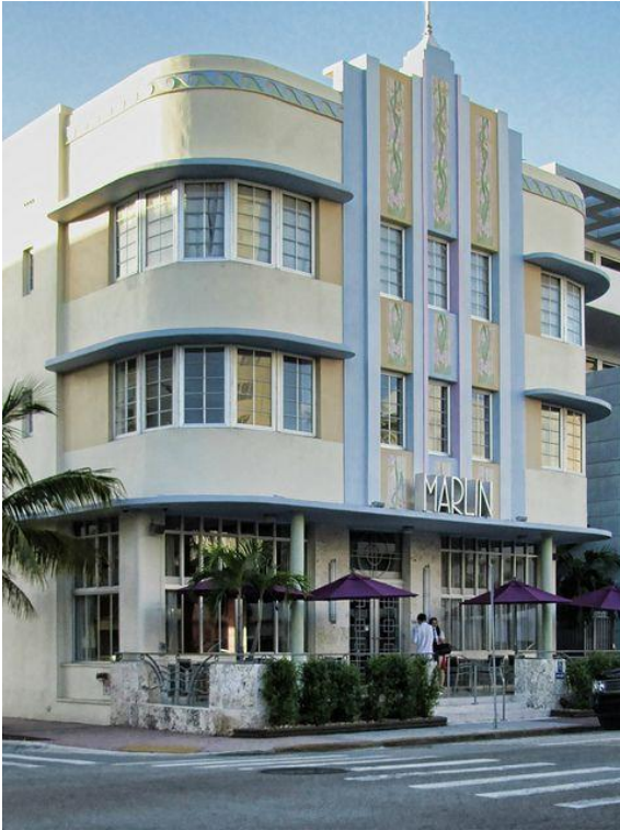
Figure 38. Marlin Hotel Source: Miami Beach, FL, Google Maps
