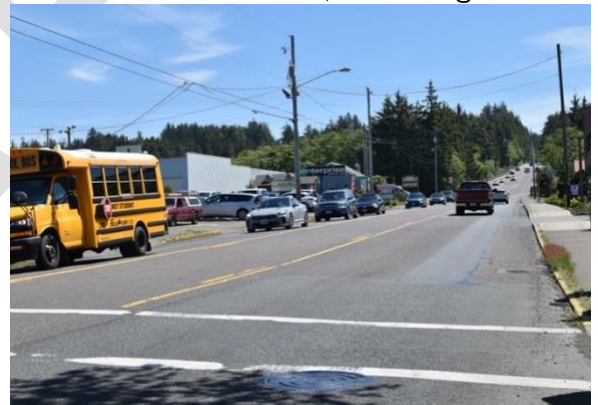
Narrow sidewalks along US 20. Crosswalk at NE Eads Street and US 20 crossing three lanes.
