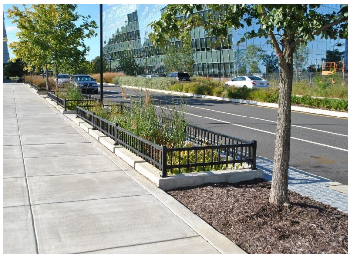
Figure 42. Streetscape Stormwater Infrastructure
