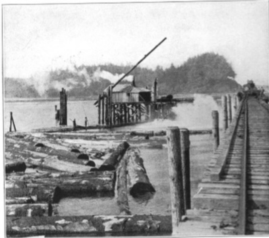
THIS VIEW SHOWS THE LOGS AT THE DUMP FROM THE OUTER END WHERE THEY ARE THROWN INTO YAQUINA BAY AND ALSO THE UNLOADING SHED AND ELEVATED "PILE" WHICH CARRIES THE LINE ABOVE THE LOGS
