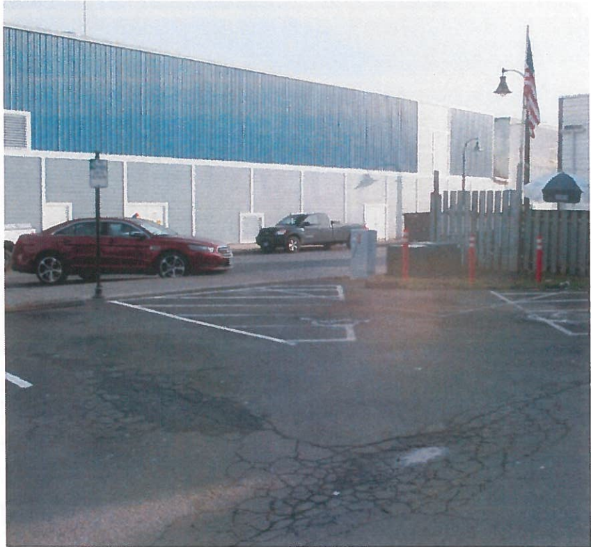
Fatigue Cracking – Abbey Street Lot (2016)
