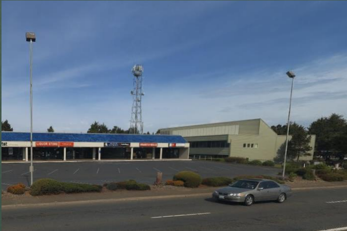
Central Lincoln Lattice Tower
