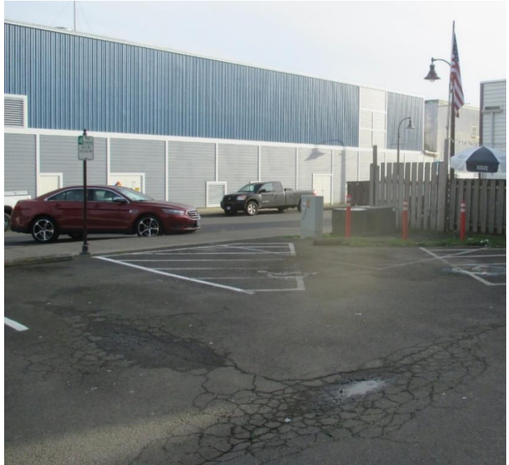
Fatigue Cracking – Abbey Street Lot
