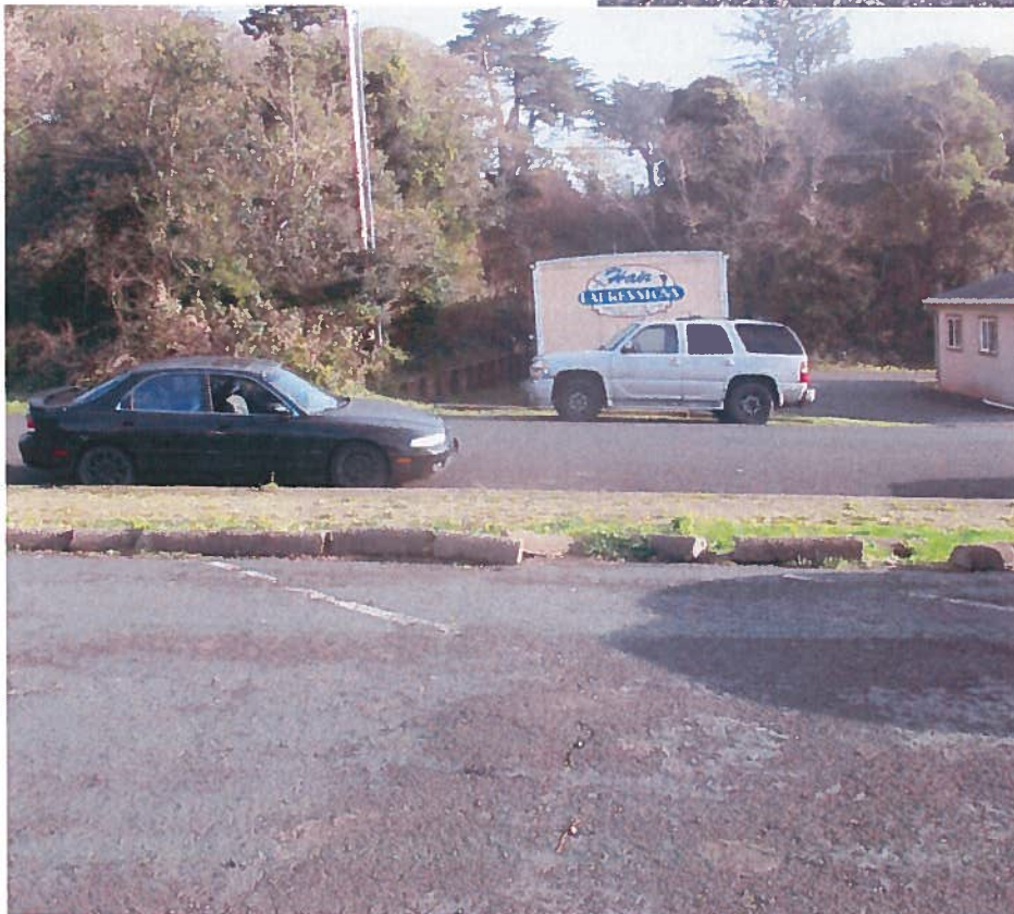
Curb Failure – 9 th and Hubert Lot
