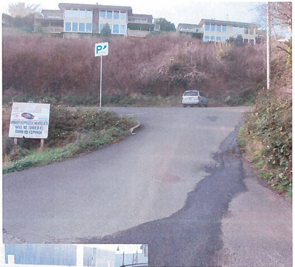
Edge Cracking – Lee Street Lot
