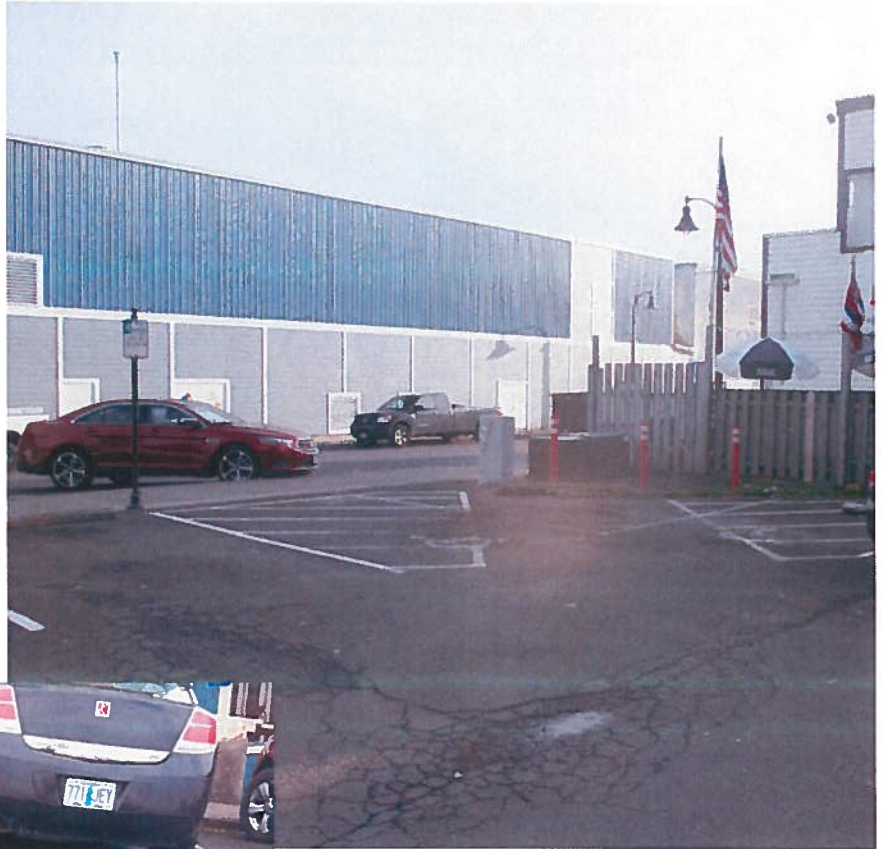
Fatigue Cracking – Abbey Street Lot
