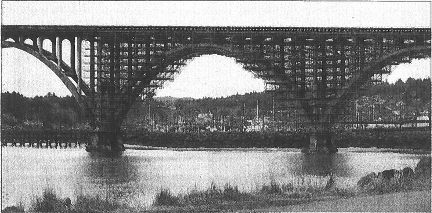
**Scaffolding covers the Yaquina Bay Bridge** as Oregon Department of Transportation contractors continue a multi-year project to replace protective coating, repair damaged concrete and install seismic upgrades. The department expects the \$30 million project will extend the bridge's life through the duration of Newport's transportation system plan currently in development, in which the bridge's future and capacity are key considerations. (Photo by Mathew Brock)
