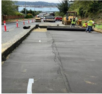
Seepage Repair John Moore Drive
