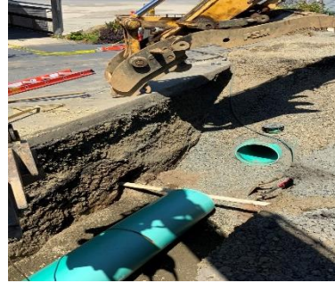
Storm Drain Replacement NW Spring St.
