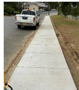
New Sidewalk Construction Harney St.
