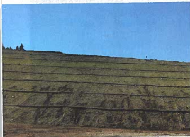
ODOT used ryegrass with straw wattles every 20 feet and geogrids every 10 feet for exposed slopes around the roadway.
