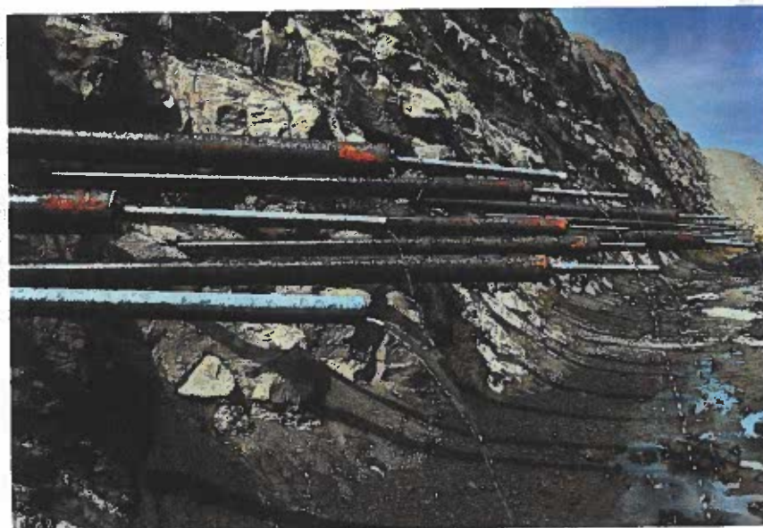
The project employed over 113 miles of horizontal drains, blanket drains, trench drains, slope ditches, and under drains during construction.
