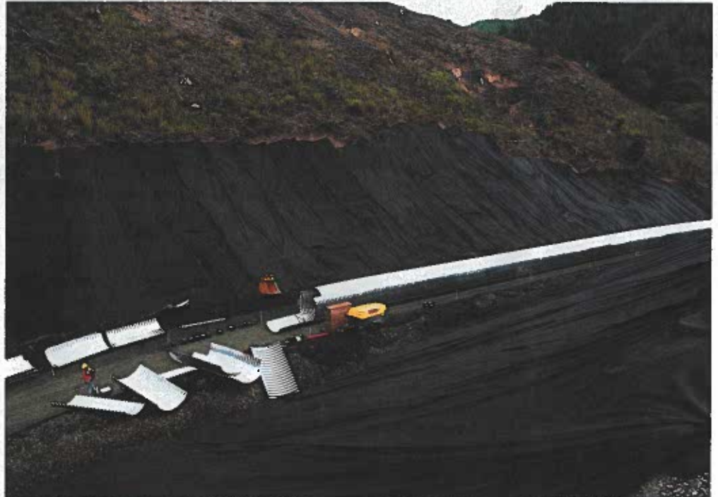
In 2013, ODOT installed 3,216 feet of culvert to keep the area's land stable.
