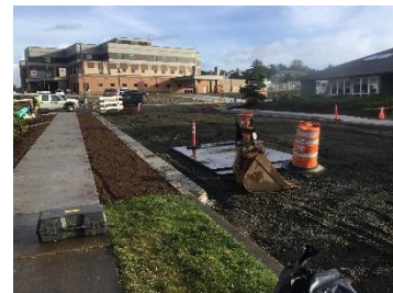
SW 9 th and 10 th Street Project
