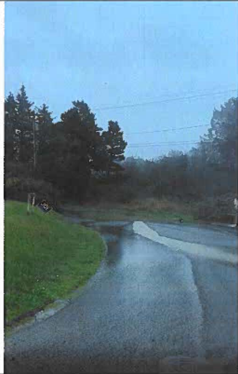
November 3, 2020 – during rain, combined runoff to NE 54 th St.
