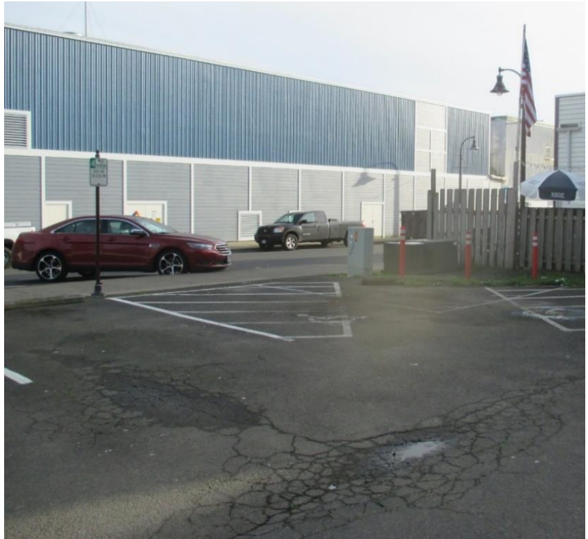
Fatigue Cracking – Abbey Street Lot (2016)
