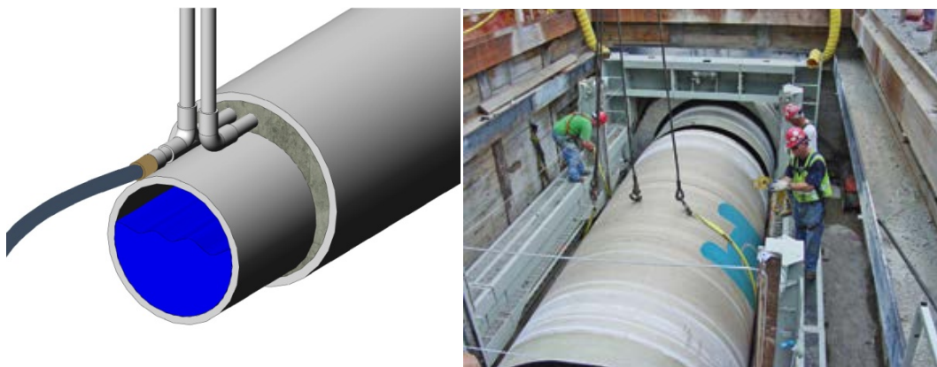
Figure D-4. Examples of sliplining installation
