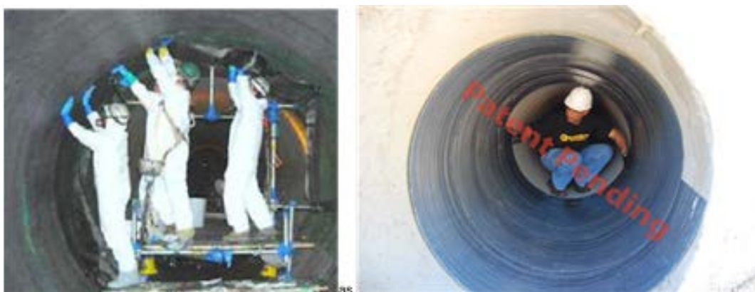
Figure D-5. Examples of pipe wrap installation
