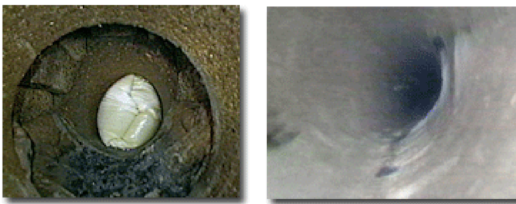
Figure D-6. Examples of cured-in-place point repair
