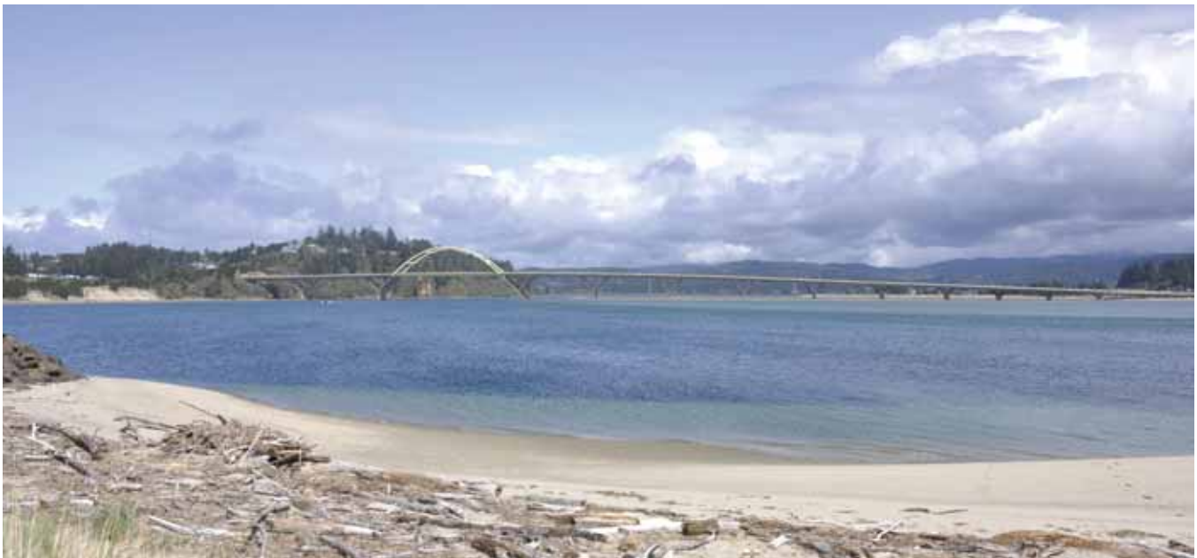
View of the Alsea Bay Bridge and Waldport River Estuary
