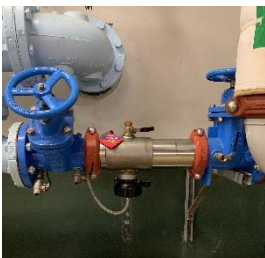
Wastewater Plant Backflow and Pipe Supports Replacement
