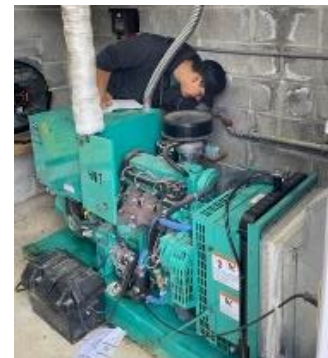
WWC crew checking lift station generators
