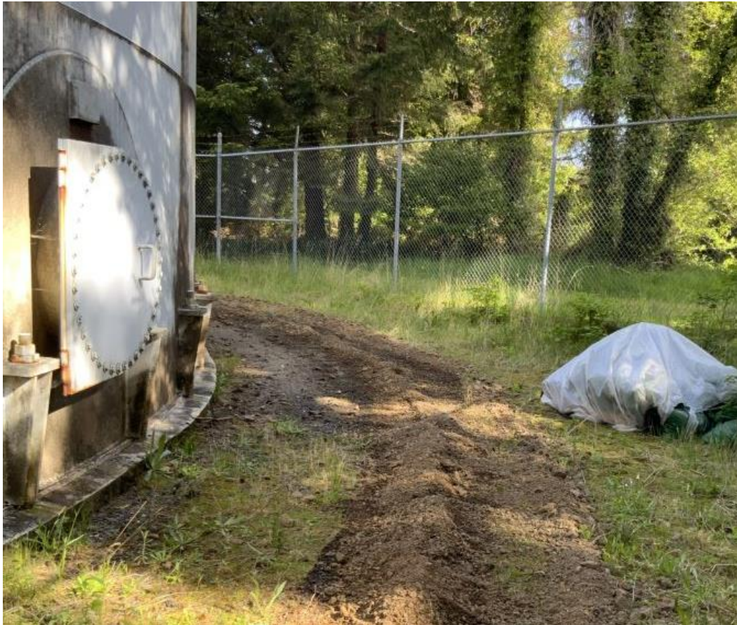
Cathodic Protection at Yaquina Heights Tank
