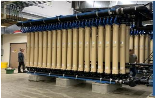
Water Treatment Plant New Filtration System
