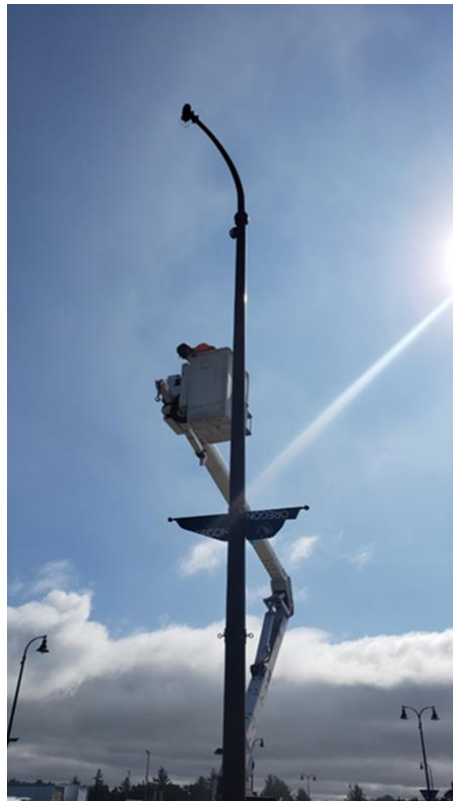
Facilities Crew Replacing a Street Light Ballast
