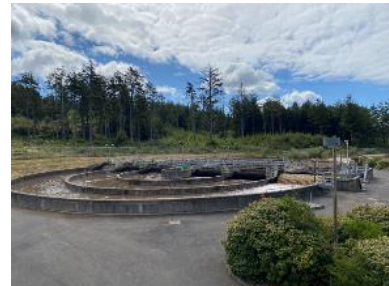
WWTP Aeration Basin
