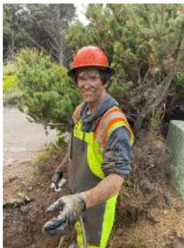
WWC crew using the Jetter
