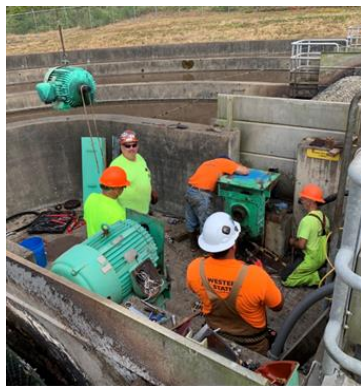
WWTP Crew Replacing the Aeration Basin Equipment
