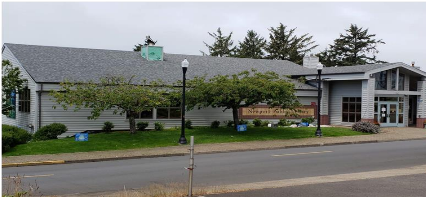
Library Roof Replacement
