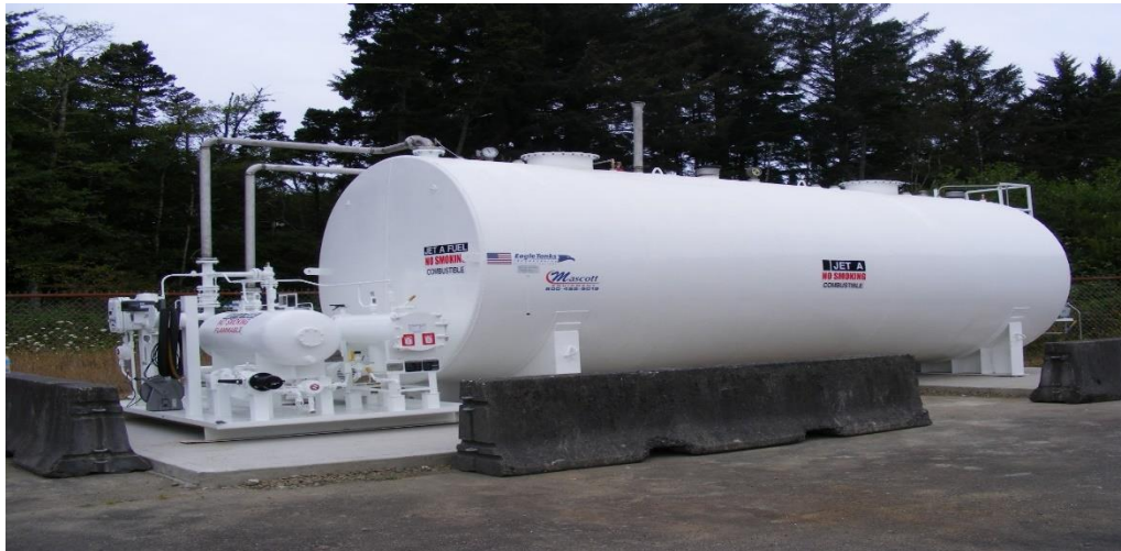
Jet A 12000 Gallon Fuel Tank- Airport
