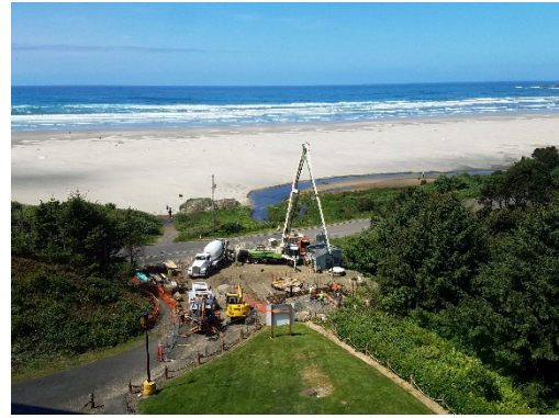
Construction Site – Agate Beach Pump Station
