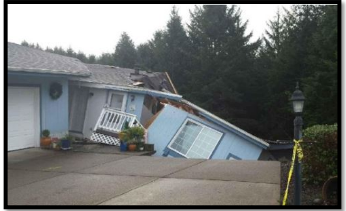
NE 70 th Street landslide
