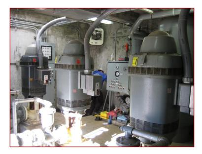
There are three pumps located within the Siletz intake. Each pump has a 200 horsepower, 460-volt, 3-phase, 1800-rpm vertical motor manufactured by U.S. Motors. Each pump is a Fairbanks Morse 12M, 7-stage, CT head vertical turbine pump rated for 1000 gpm at 560 feet total dynamic head (TDH). With two pumps running at once the station output is approximately 2200 gpm with a discharge pressure exceeding 200 psi.
