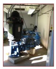
The finished water service pumps are located in the lower level of the water treatment plant. Different combinations of pumps are operated depending on the desired throughput of the water plant. The following finished water pumps are currently utilized in Newport:
