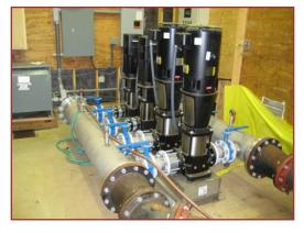
The station equipment is a Grundfos Booster PAQ with on/off control based on pressure in a hydro-pneumatic tank located inside the building. Power supply is 460 volt, 3 phase. Four
