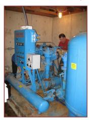
Suction pressures range from 40 to 47 psi depending on pumping rate and water level in the Main Storage Tanks. Discharge pressure of 80 psi in the pressure tank (HGL = 350') provides a pressure of about 52 psi at the top of the service area (elev. 230'  $\pm$ ). The service area is relatively small and is unlikely to increase in size unless service outside the UGB is provided in the future.
