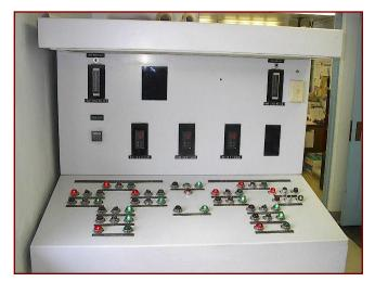
An online chlorine analyzer monitors the chlorine levels in the clearwell. The chlorine dosage rates are manually adjusted based on the feedback from the analyzer.
