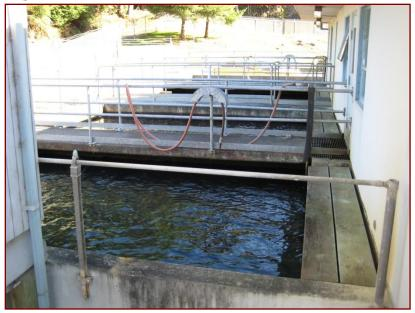
propagate into the clay underdrains. The filter has consistently experienced short circuiting and turbidity break through as a result of the damaged under-drain system. Replacement underdrain tiles that match the existing tiles are not readily available today.
