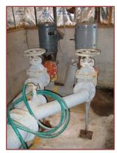
pressure zone and boosts pressure for the surrounding small neighborhood. The station contains two 10 Hp Cornell close coupled centrifugal pumps that were relocated from an older pump station. An associated pressure tank is located at the top of Lakewood Drive at a ground
