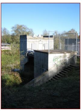
needs. Small solids handling pumps could be added to facilitate silt removal prior to summer pumping. Shut-off valves or gates to isolate the wetwell from the river cannot be added since a flooded wetwell is required to prevent uplift during high river conditions.
