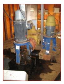
The pumps are low head pumps that lift the water a short distance to the nearby Big Creek treatment plant.
