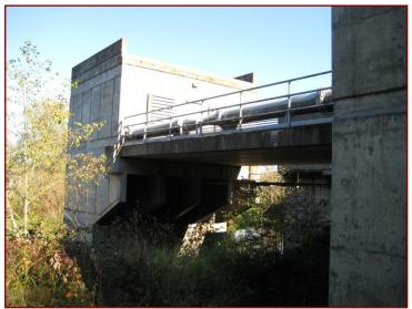
pipe was installed to connect the intake to the upper Big Creek reservoir. Velocity in the 16-inch transmission piping at the full water right of 6 cfs (2693 gpm) is 4.3 feet per second.
