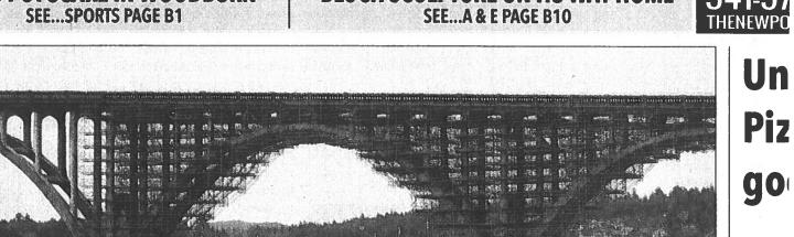
Scaffolding covers the Yaquina Bay Bridge as Oregon Department of Transportation contractors continue a multi-year project to replace protective coating, repair damaged concrete and install seismic upgrades. The department expects the \$30 million project will extend the bridge's life through the duration of Newport's transportation system plan currently in development, in which the bridge's future and capacity are key considerations. (Photo by Mathew Brock)
